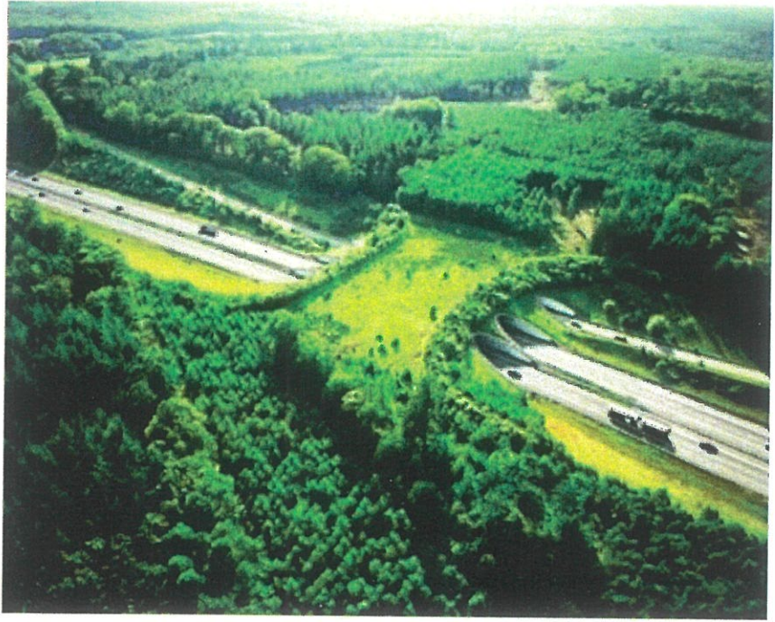
Viaduct for animal overpass ( https://www.youtube.com/watch?v=U6lWv8enIAw )
