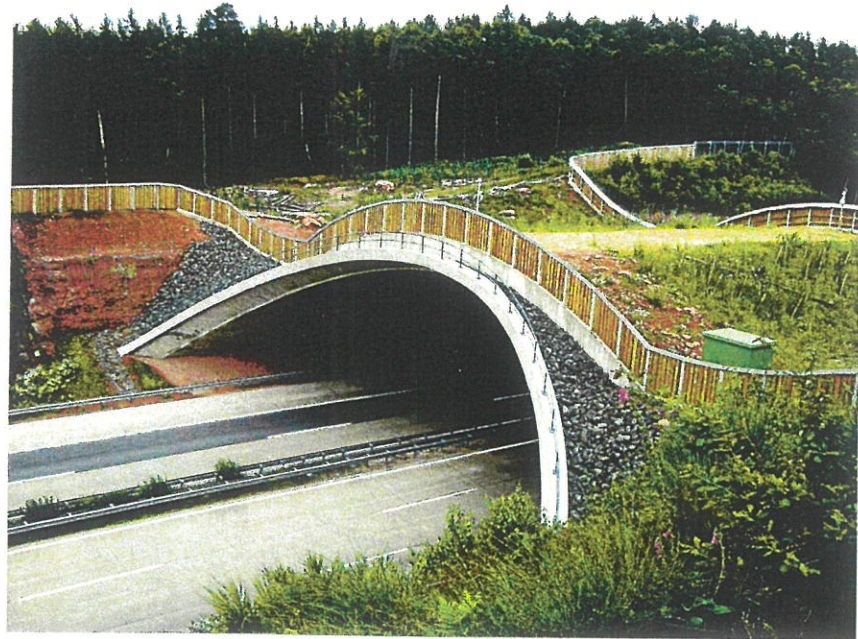
Viaduct for animal overpass with guided fence
